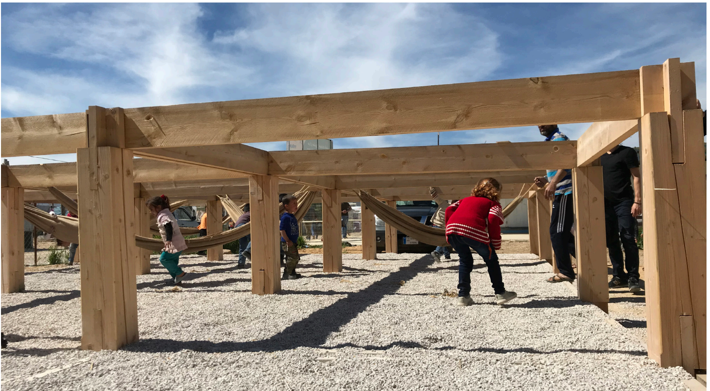
Figure 14: Once deemed safe, and outside of working hours, children began to use the playground only days after construction began. Here they enjoy the modular system itself as a full sized play structure, also playing and gathering around low hanging hammocks.
