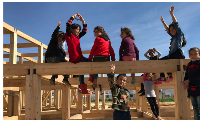
Figure 16: Children gather in the space, testing the structure and enjoying an elevated view of the Bekaa.
